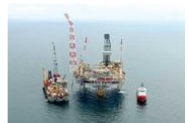
The Shah Deniz TPG 500 platform installed and jacked up to operational position
